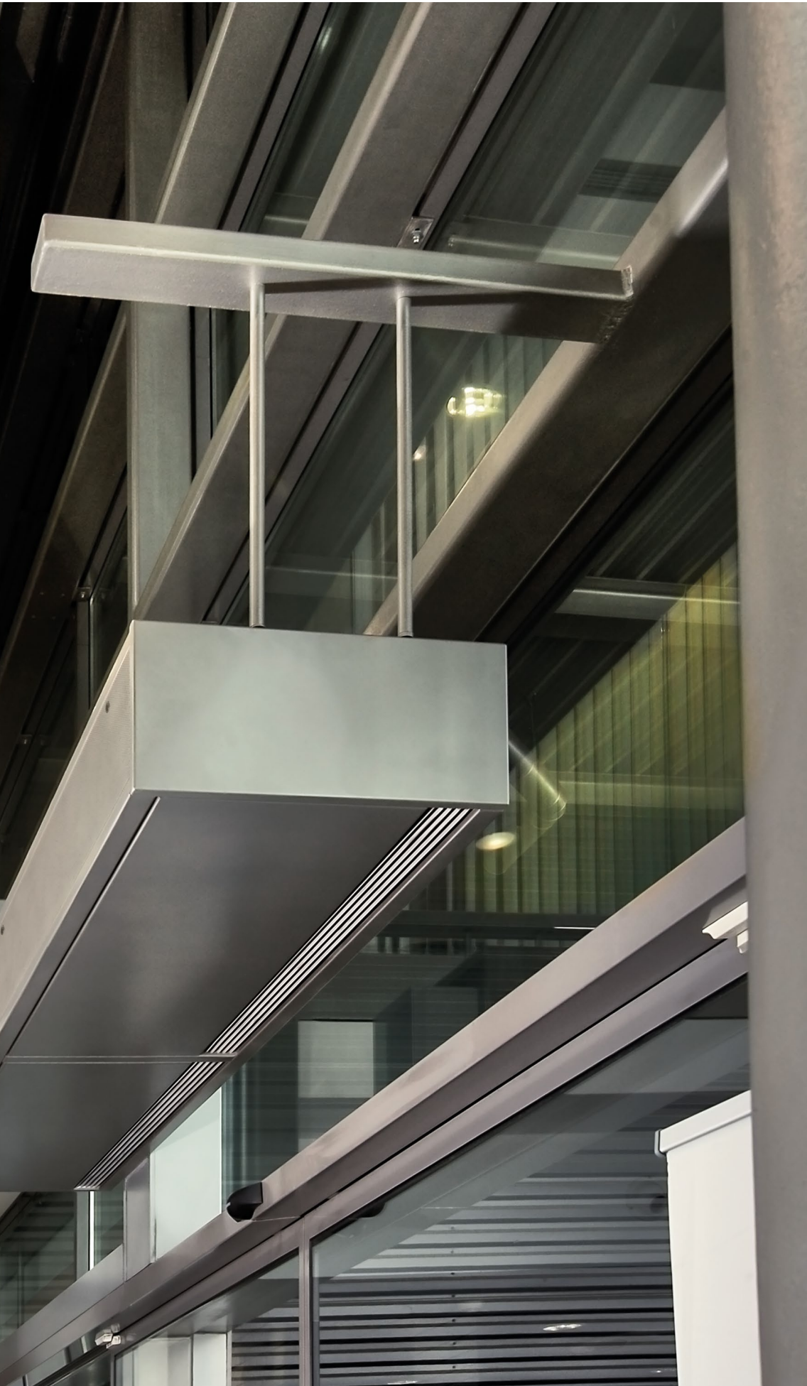
Porsche Centre, Moscow: The screening effect of UniLine door air curtains effectively counters heat losses and produces a comfortable interior climate.
