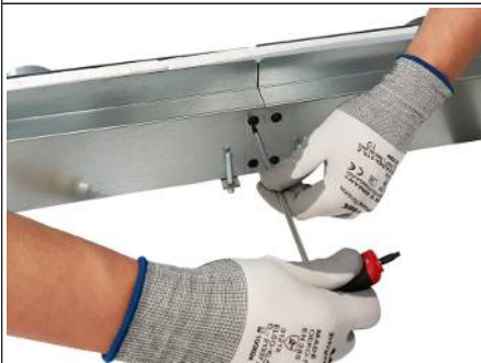
Fig. 7: Screwing the plenum boxes together
