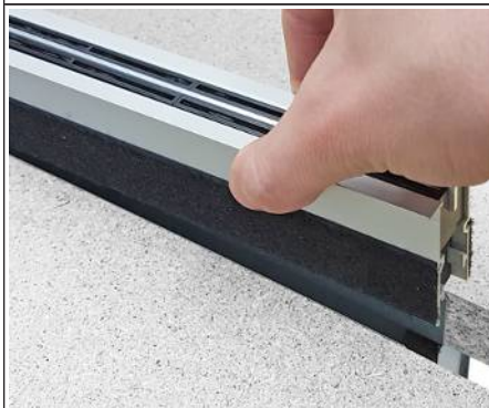
Fig. 11: Inserting the slot outlet
