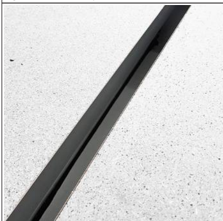
Fig. 10: Plenum box flush in the floor
